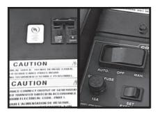
Now switch the generator's main breaker ON and put the mode switch in AUTO.
